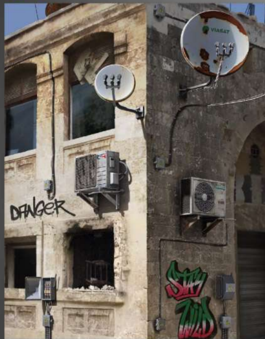
35638 AIR CONDITIONERS & SATELLITE DISHES
